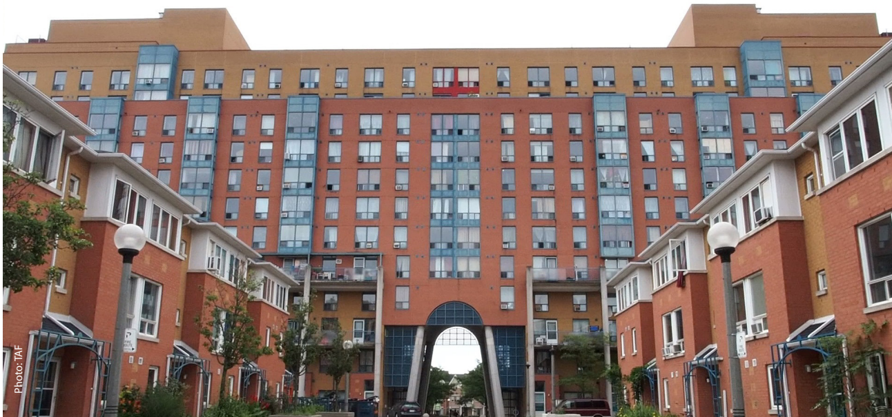
The Robert Cooke apartment co-op in Toronto received $460,000 in energy retrofits through an ESPA with the Toronto Atmospheric Fund
