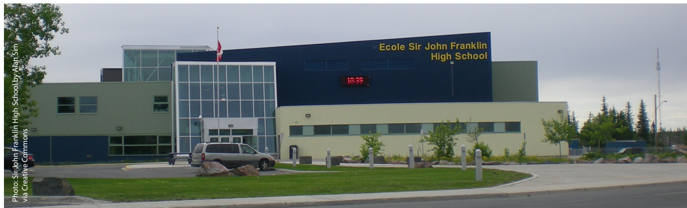
Arctic Green Energy established a successful energy service contract with the GNWT for Sir John Franklin school
