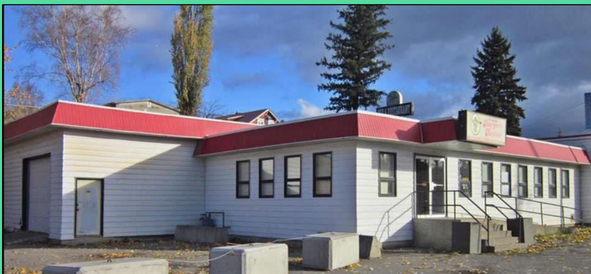
Figure 2: SKRFH building at 101 Marsh Drive, West Quesnel BC (SKRFH, n.d.)
