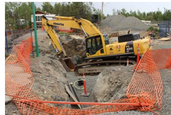
Northlands infrastructure upgrades (City of Yellowknife Photo)
