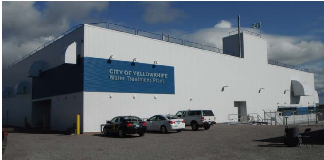
Photo: Outside, front view of the Water Treatment Plant.
