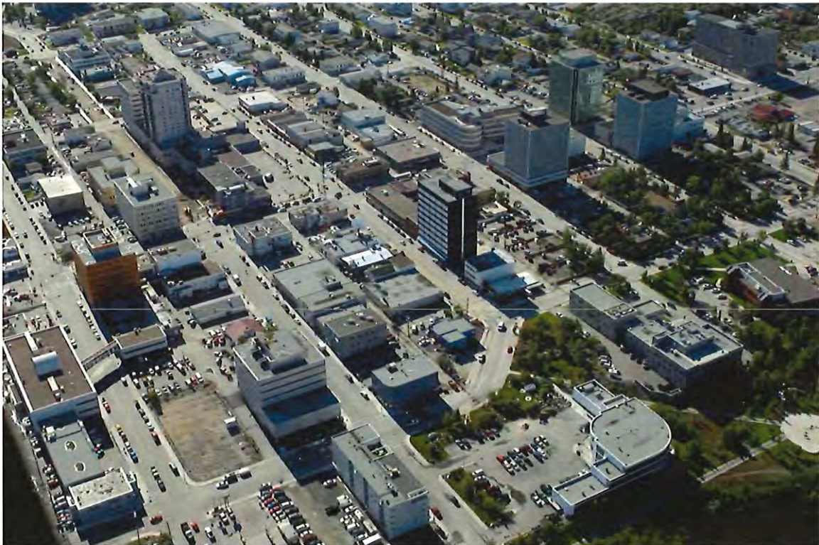
Exhibit 5-4: Overview of Downtown and Parking
