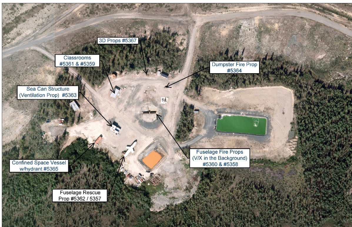
Image 4: Fire Training Facility Props and Structures
