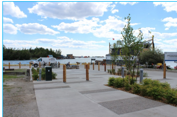
Paving, landscaping and bike racks were among the additions to the Government Docks. City of Yellowknife photo.
