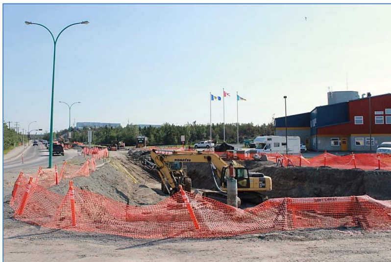
Corrugated metal pipe replacement along Franklin Ave. City of Yellowknife photo.
