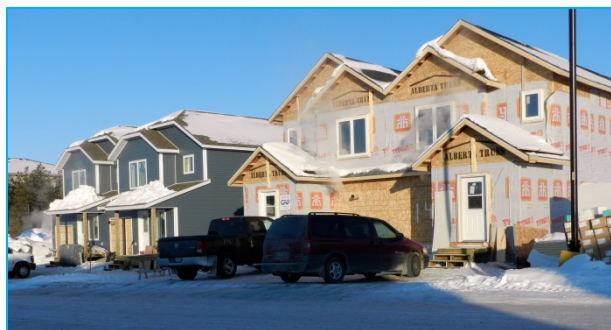
Single-family unit construction in Niven Lake. City of Yellowknife photo.
