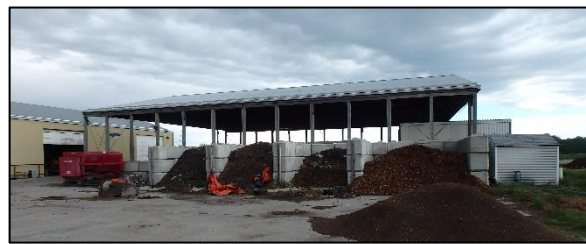
FIGURE 2 AERATED COMPOSTING BUNKERS IN OLDS, ALBERTA BUILT FROM PRE-CAST CONCRETE BLOCKS
