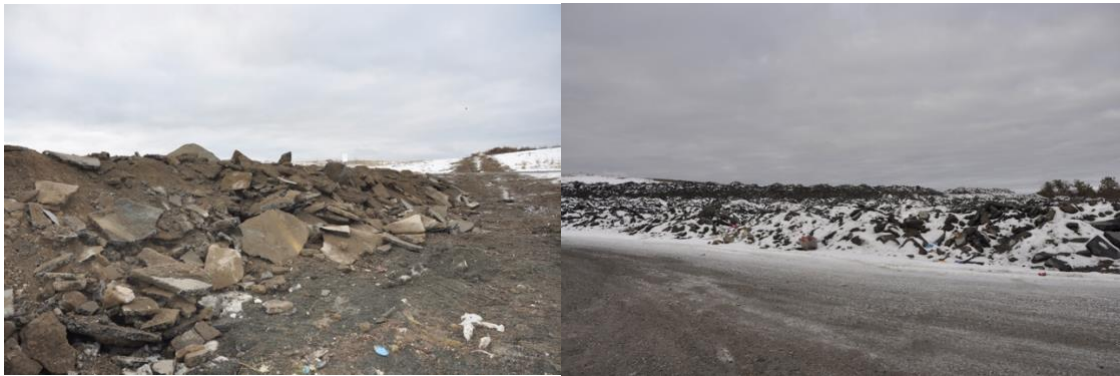
Figure 72: Asphalt Piles for Diversion
