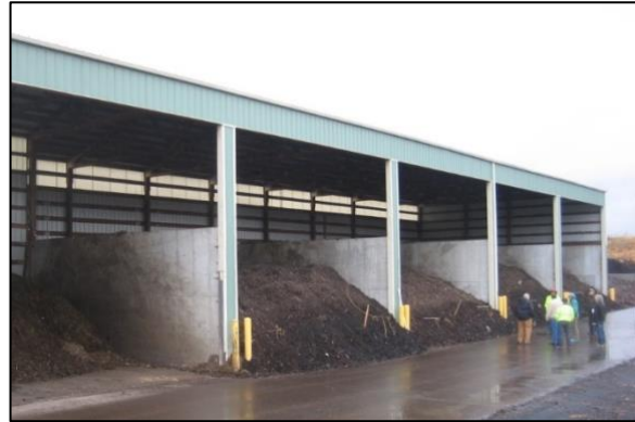
Figure 79: Aerated Composting Bunkers in Moscow, Idaho, with Wood Frame Roof Structure
