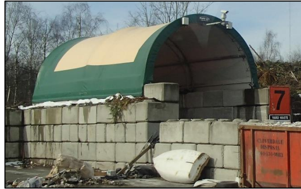
FIGURE 5 ENCLOSED WASTE RECEIVING BUNKER
