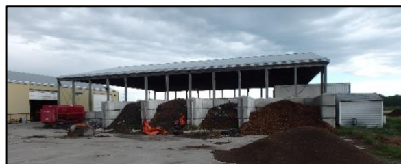
Figure 78: Aerated Composting Bunkers in Olds, Alberta built from pre-cast concrete blocks
