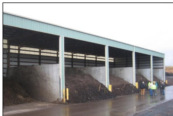
FIGURE 3 AERATED COMPOSTING BUNKERS IN MOSCOW, IDAHO WITH WOOD FRAME ROOF STRUCTURE
