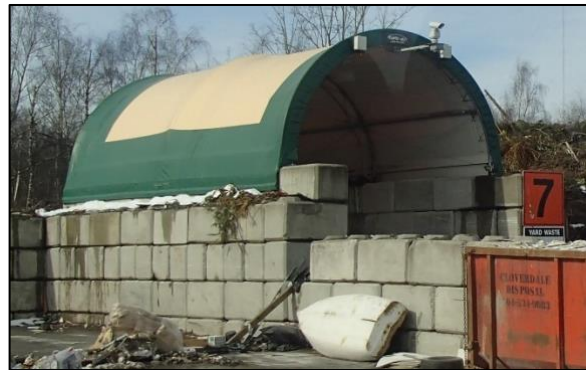
Figure 81: Enclosed Waste Receiving Bunker
