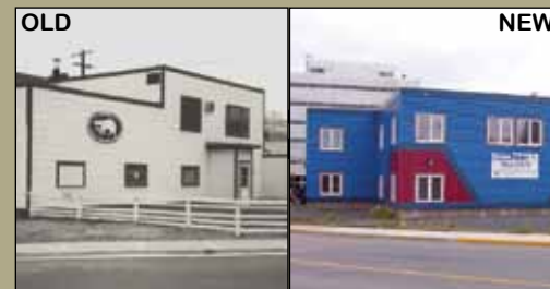
OLD MINE RESCUE STATION (4903 50th Street)
