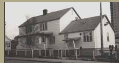
RCMP STATION (5019 51st Street)
