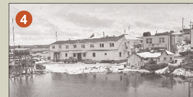
4 Old CPA Office This building celebrates the role of the floatplane companies and their adventurous pilots. It was built in 1946 and used as office and staff housing for many years by various charter companies, including Canadian Pacific Airlines. At one time in the 1990s, it housed Yellowknife's first brewing enterprise and had a long bar fashioned from an aircraft wing.
