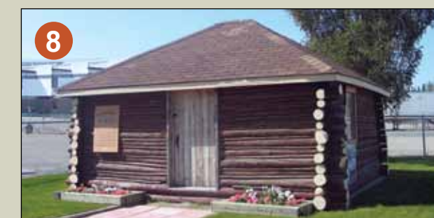
8 Mildred Hall Schoolhouse The original Yellowknife school is one of the more notable heritage buildings. Built in 1937 by a mining company, it was rented to the local Trustee Board and used as a schoolhouse for a short period before World War II. Mildred Hall was the teacher, whose name is also commemorated on the modern elementary school.
