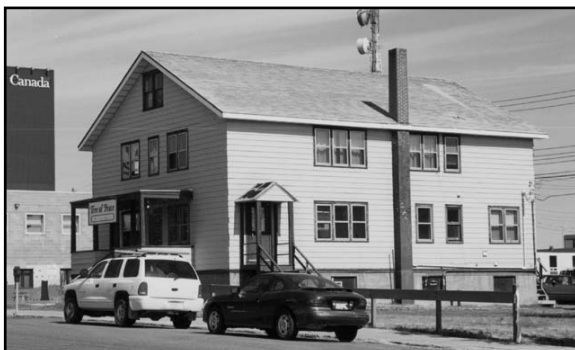
The Old Federal Building - Demolished 2005
