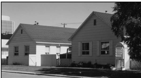
Department of Transport Houses
