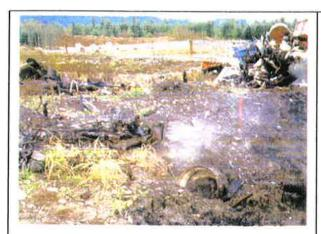
Photo 9-3 Smoke and Cracking in Soil Cover Terrace, B.C.
