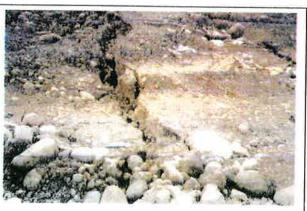
Photo 9-11 Major Settlement crack Due to Fire
