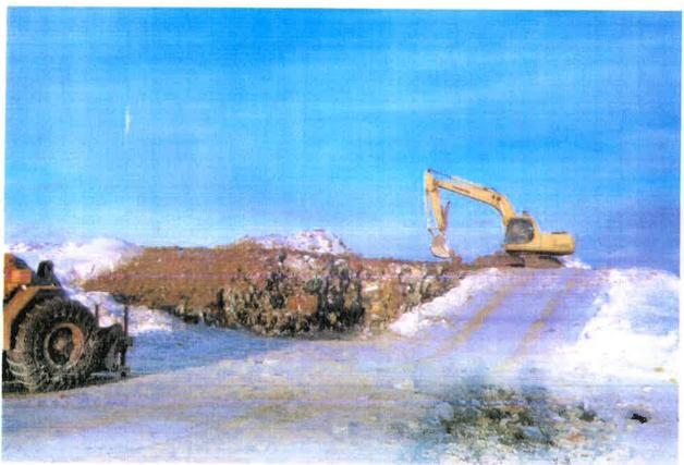
Photo 11-9 Intermediate Cover Fire Wall being placed at Colechester Bale Fill, N.S.
