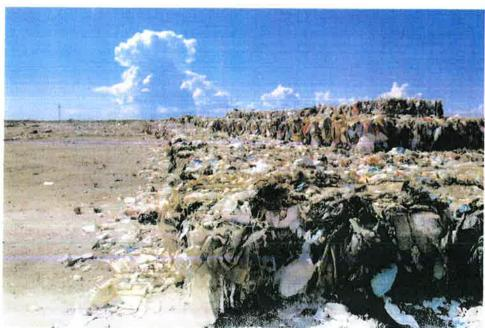
Photo 11-7. MSW Bales stacked without proper cover at Yellowknife
