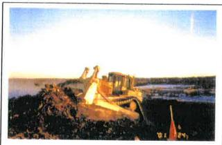
Photo 8-10 Suppressing Oxygen with Dirt. C & D
