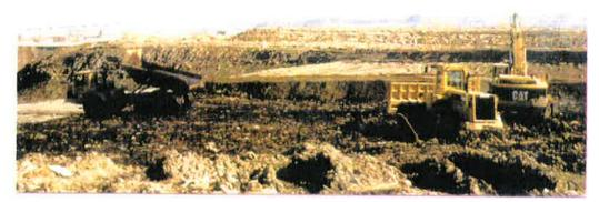
Photo 11-8 Encapsulated Cell Under Construction at Delta Shake
