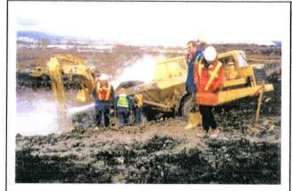
Photo 8-14 Excavating C & D Waste at Delta
