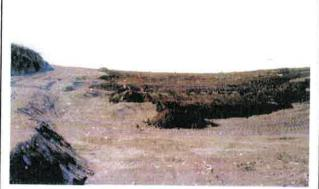
Photo 8-13 Topsoil placed on clay barrier to prevent desiccation cracking, Penticton B.C Fire.
