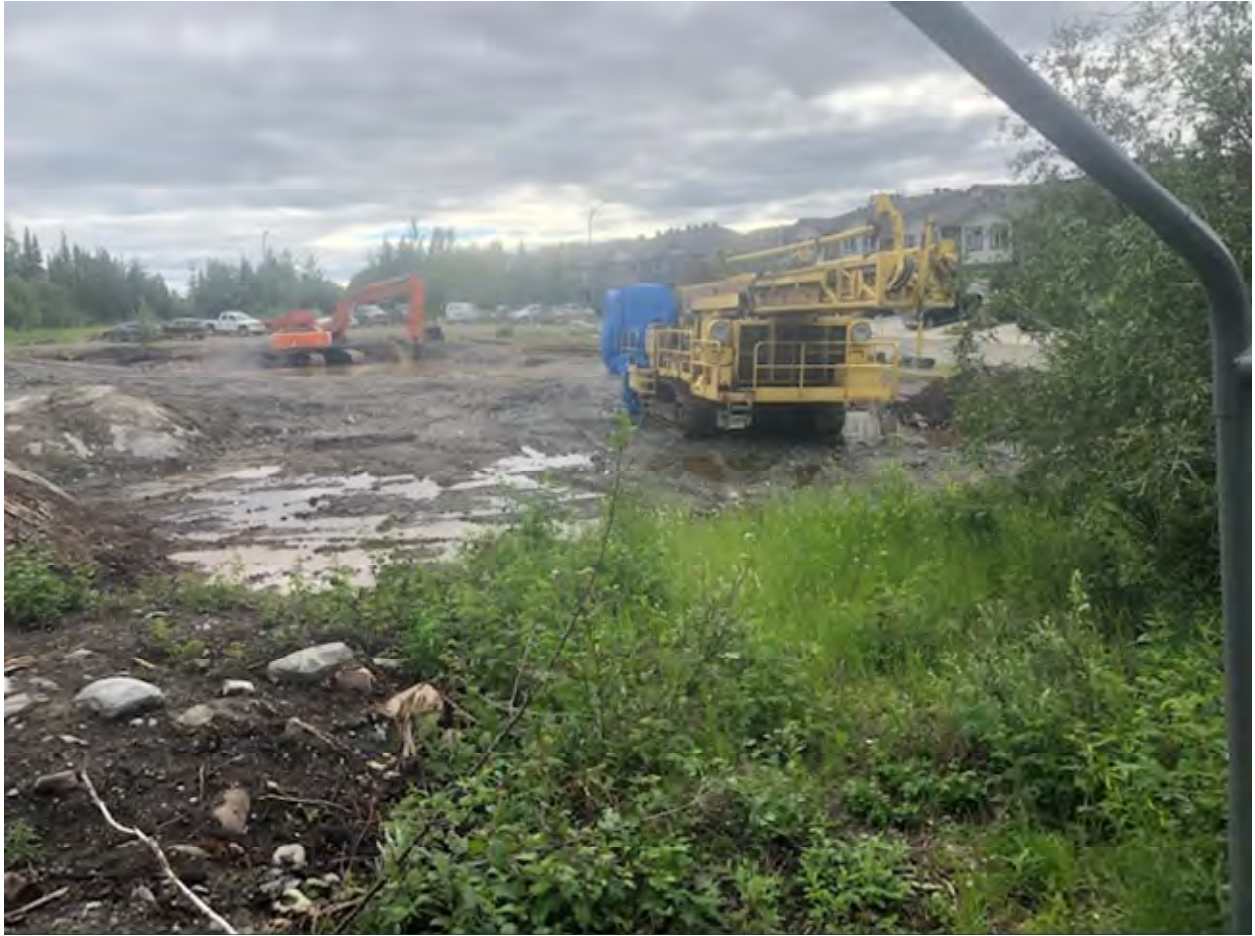
July 15, 2020 – Over-all site clearing
