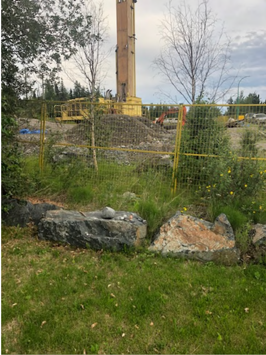
July 19, 2020 – Build up of pad, over .6 m
