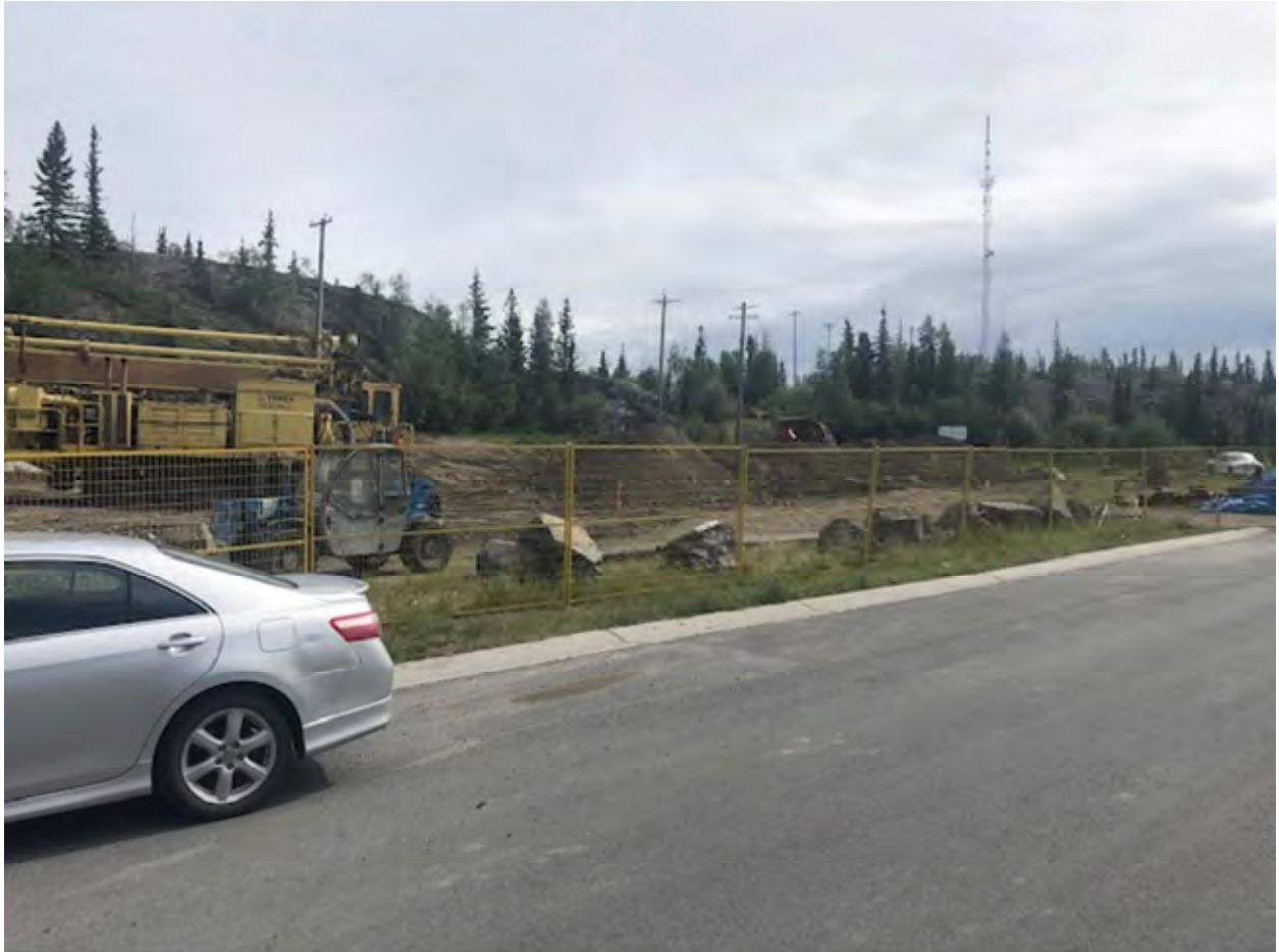
July 9, 2020 – Excavation and grading over .6 m
