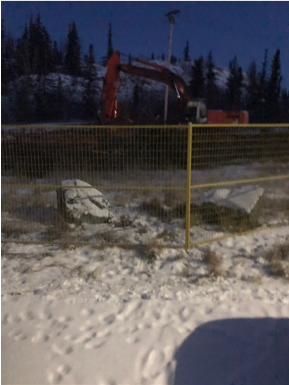
November 13, 2019 – Excavation and grading start
