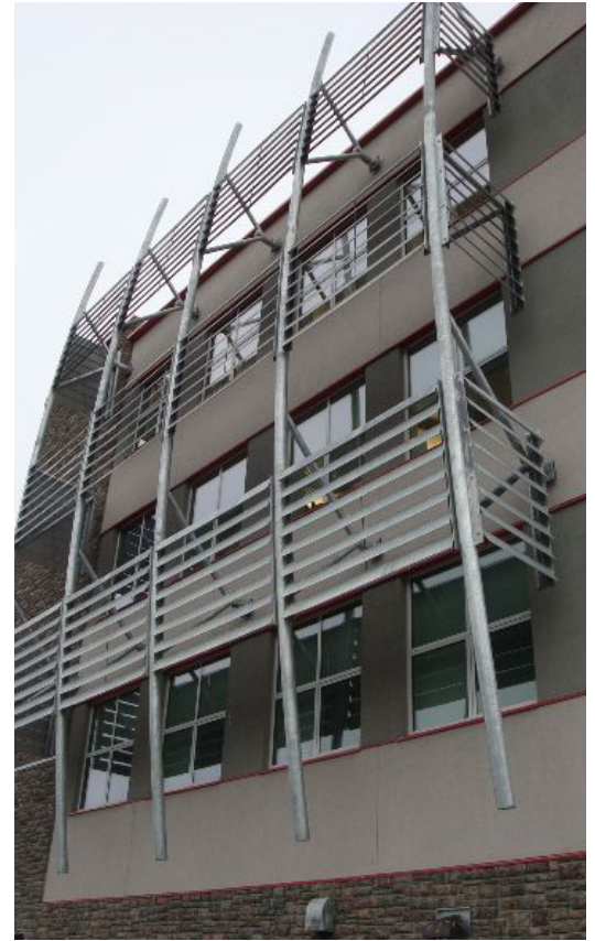
These sun louvers on the Greenstone building in Yellowknife let the sun in at certain times of year, while blocking it at others. They also add architectural interest.
