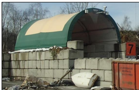
Figure 81: Enclosed Waste Receiving Bunker
