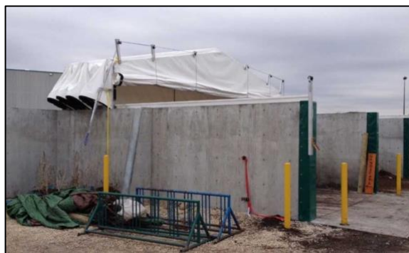
Figure 82: Aggregate bunker with RollCov-R roof system (source: Chameleon Innovations)
