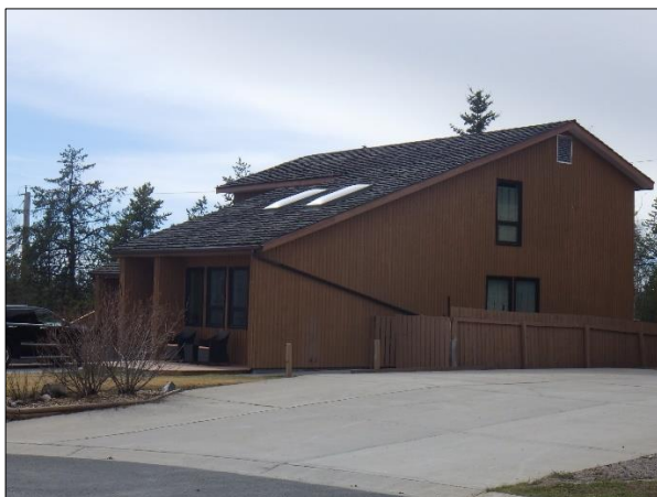
Combustible Wood-Shake Roof & Wood Siding
