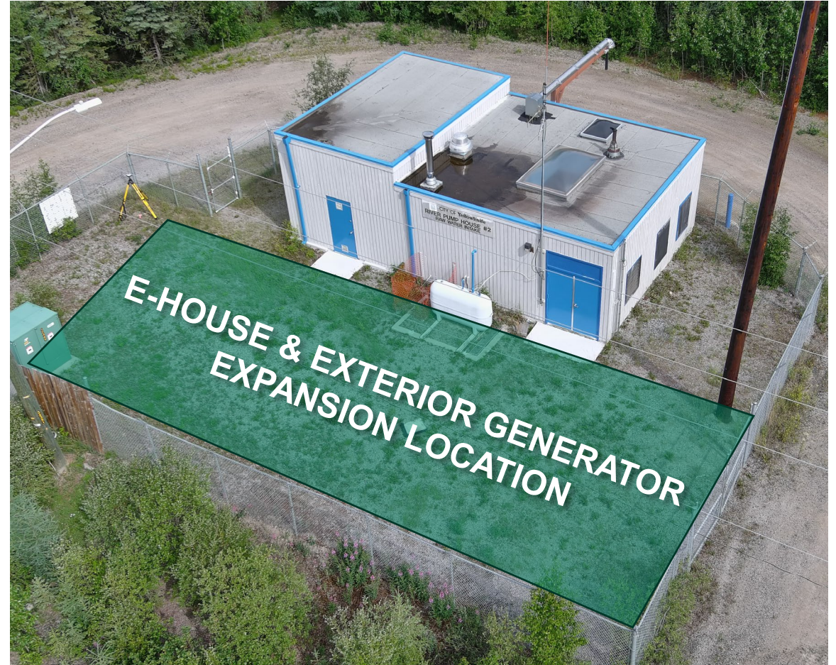
Proposed Upgrades – Pumphouse No. 2
