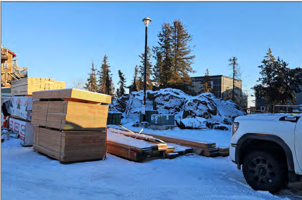
Photo 2: Outcrop at 2 Findlay Point, taken from street Dated: November 15, 2025
