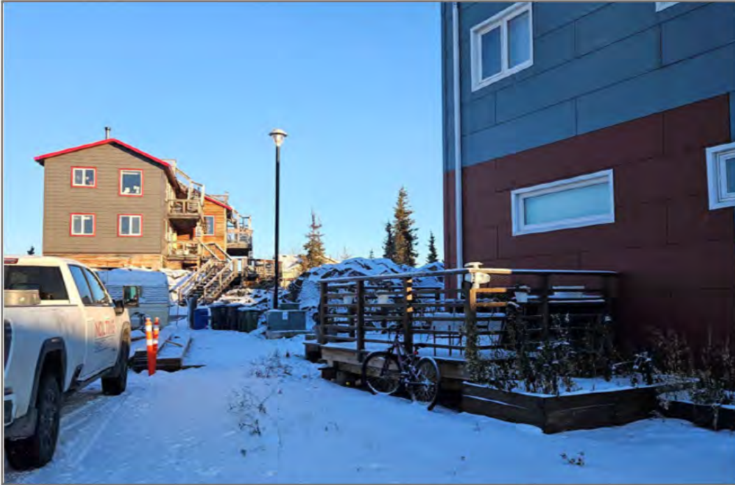
Photo 1: Street side of site, taken from corner of Findlay Point and Moyle Drive Dated: November 15, 2025
