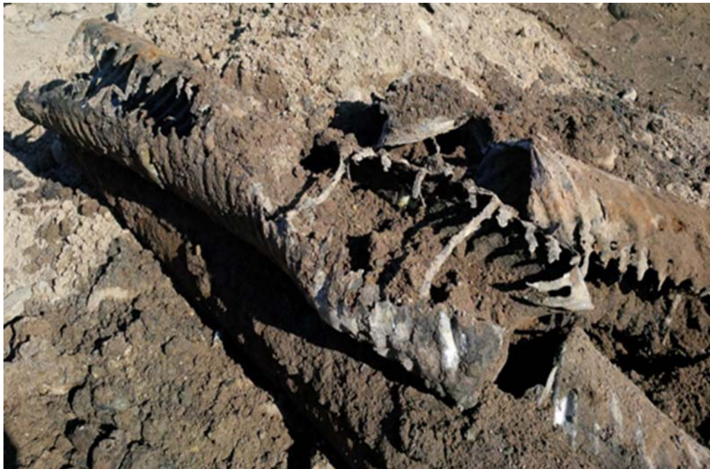
Photo: Failed CMP sewer main showing no bottom left in the pipe
