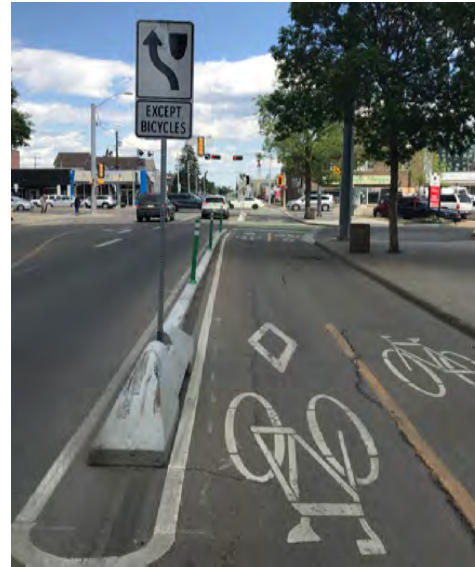
PROTECTED BICYCLE LANE CONSTRUCTED USING A RAPID IMPLEMENTATION APPROACH
