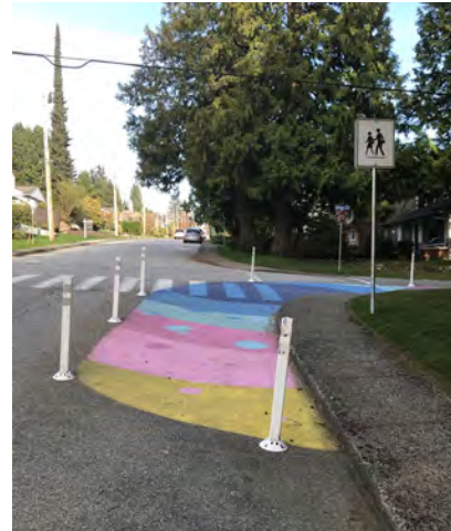
CURB EXTENSIONS IMPLEMENTED THROUGH A LOW-COST TACTICAL URBANISM APPROACH
