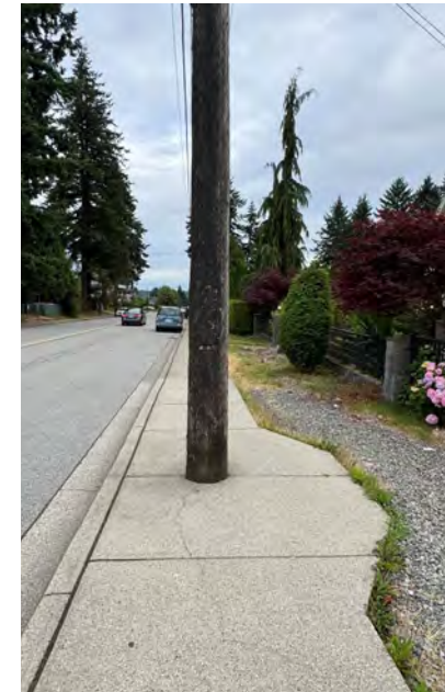
INACCESSIBLE SIDEWALK WITH OBSTRUCTION
