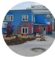
Mine Rescue Building
